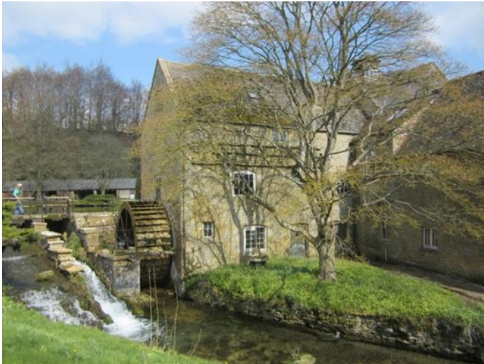
The Rear of the Brewery and Waterwheel
