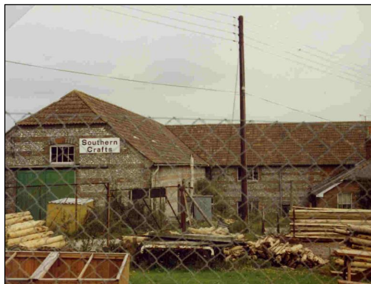
Former Durweston Brewery
